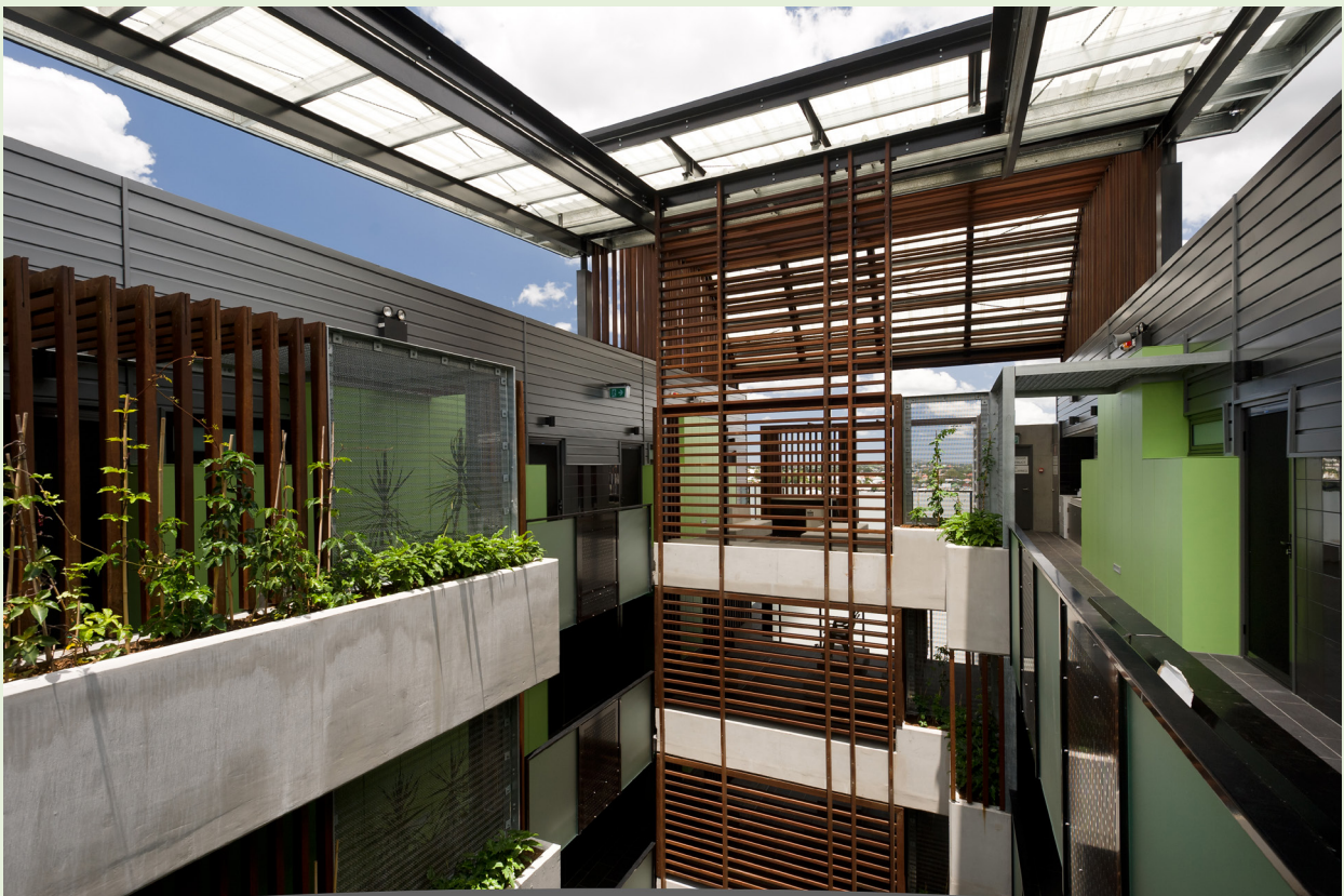
5 Green Square Close, Fortitude Valley, Queensland (Source: Brisbane Housing Company Limited)
